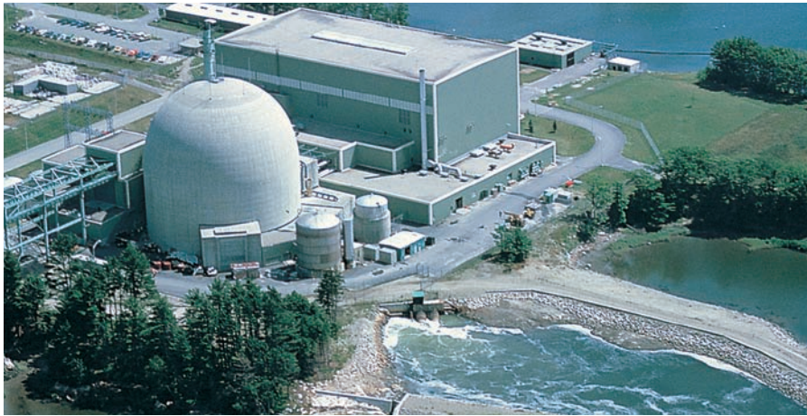
FIGURE 23.14 A light-water nuclear reactor. A , Photo of a facility showing the concrete containment shell and nearby water source. B , Schematic of a light-water reactor.
