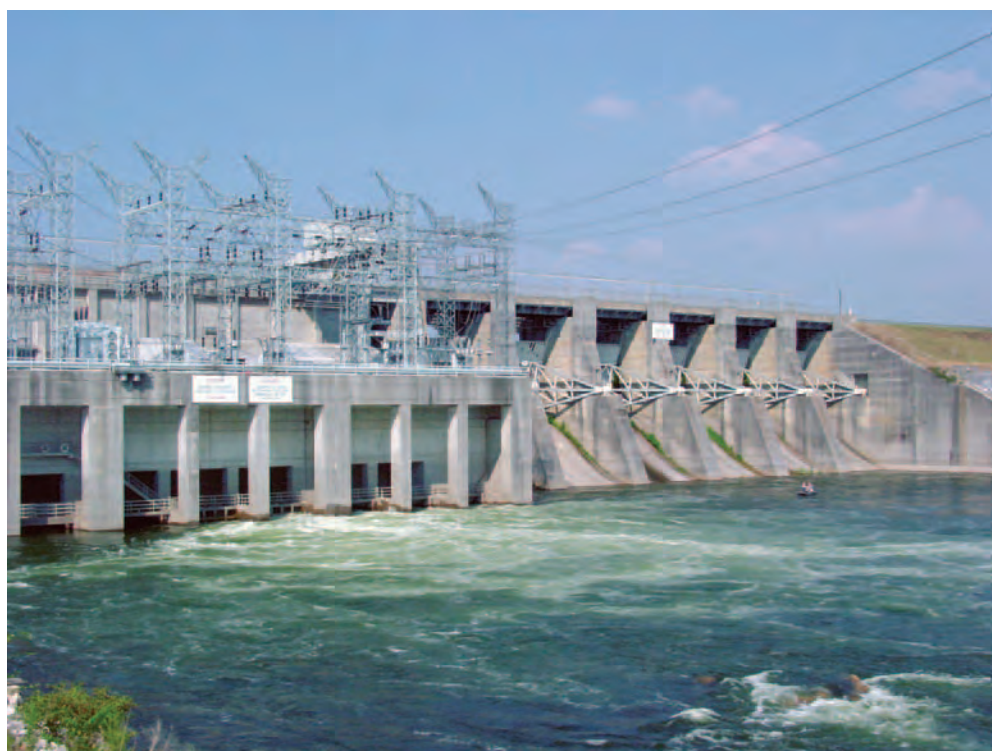
Figure 11.1 Hydroelectric generating facility. (Courtesy of Mark Nelms)
