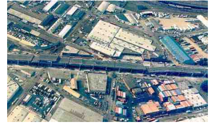
I / The collapsed section of the Nimitz Freeway
