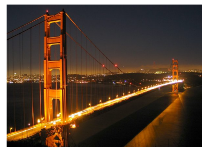
o / The Golden Gate Bridge's roadway is held up by the tension in the vertical cables.
